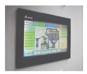
The ZAC is supplied with a full colour 10" touch screen interface to allow fine tuning of the separation process.
