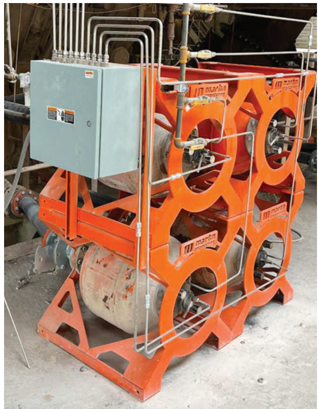
Martin® X-Stand with a solenoid box mounted on the side for better access.
