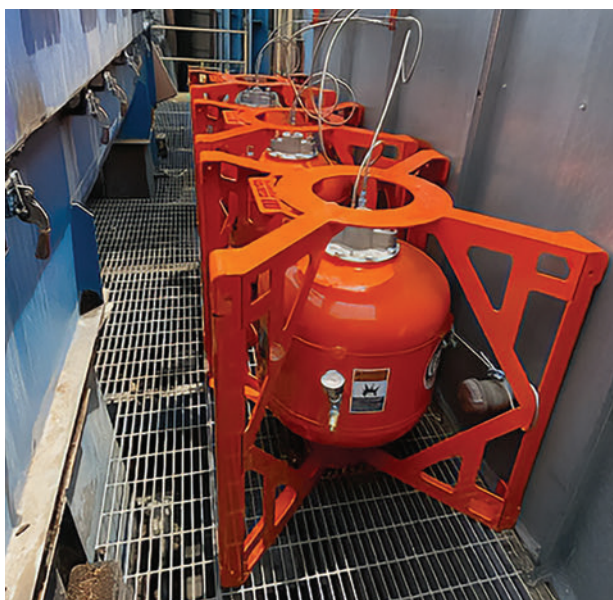
The positioning of the cannon can redirect pipes to go underneath the walkway, improving access.
