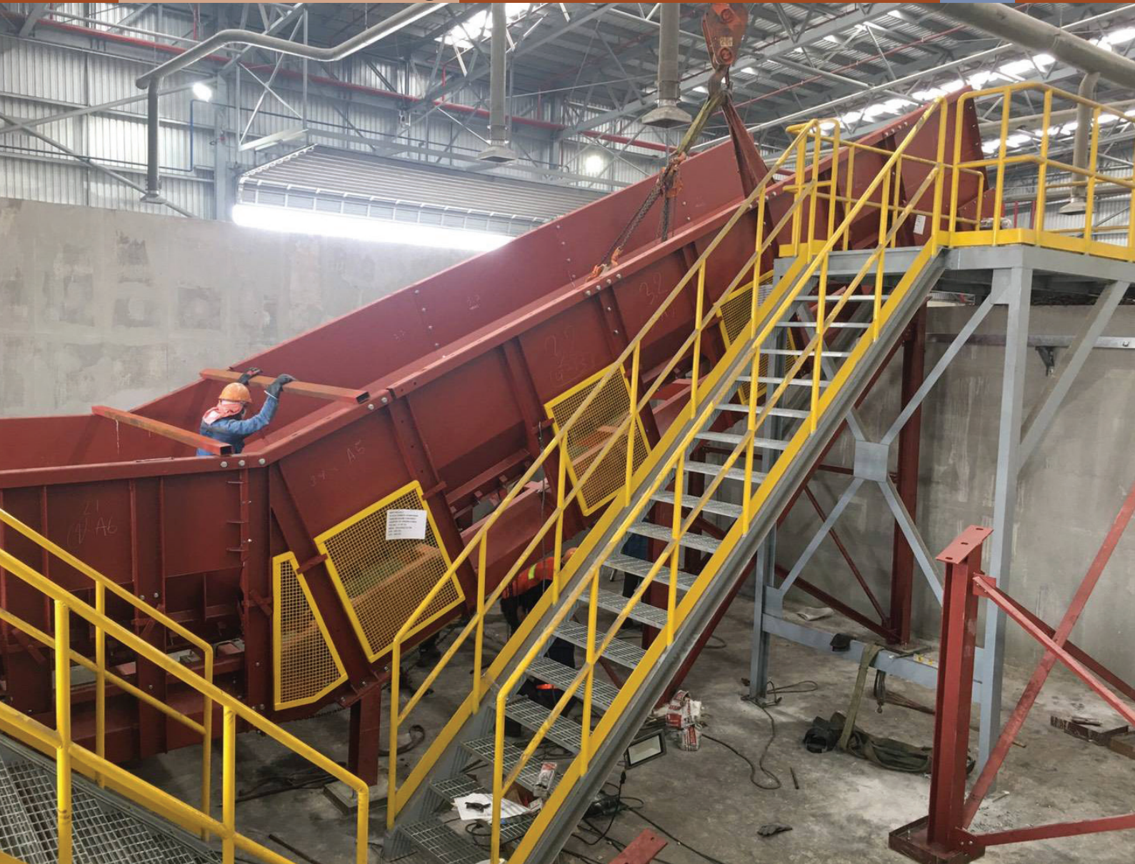
Onsite installation of the Samson Material Feeder
