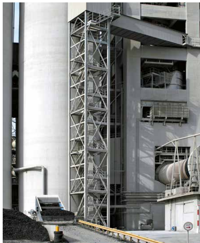
Regulated discharge with Screw Metering Feeder direct to Bucket Elevator
