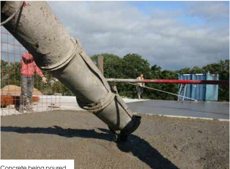
Concrete being poured
