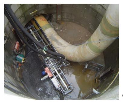
Aptech has supplied two pneumatic conveying systems as part of a major gas pipe project in the Greater London area. The systems were designed to backfill 6ft and 8ft tunnels with ground glass or sand.
