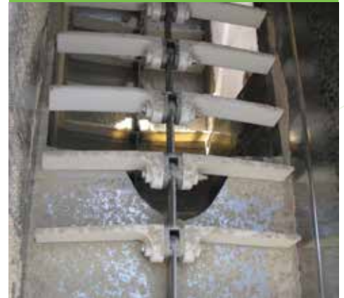
Feed Mill Application using Bolt-N-Go Chain with Nylon Flights
